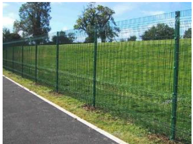
Figure 4-11 Paladin Mesh Fence
