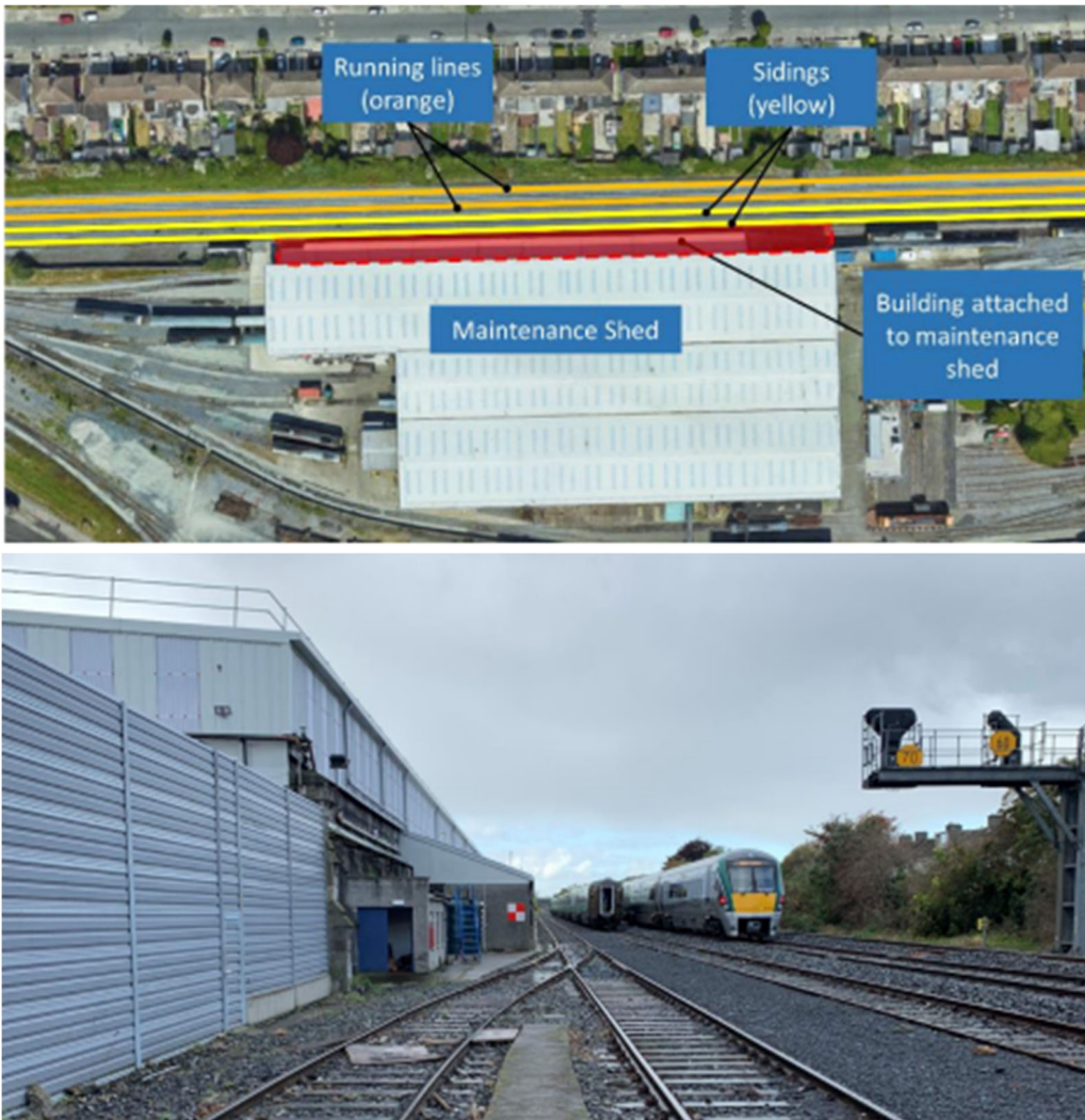
Figure 4-77 Maintenance Shed, Attached Building and Sidings, Inchicore Works
