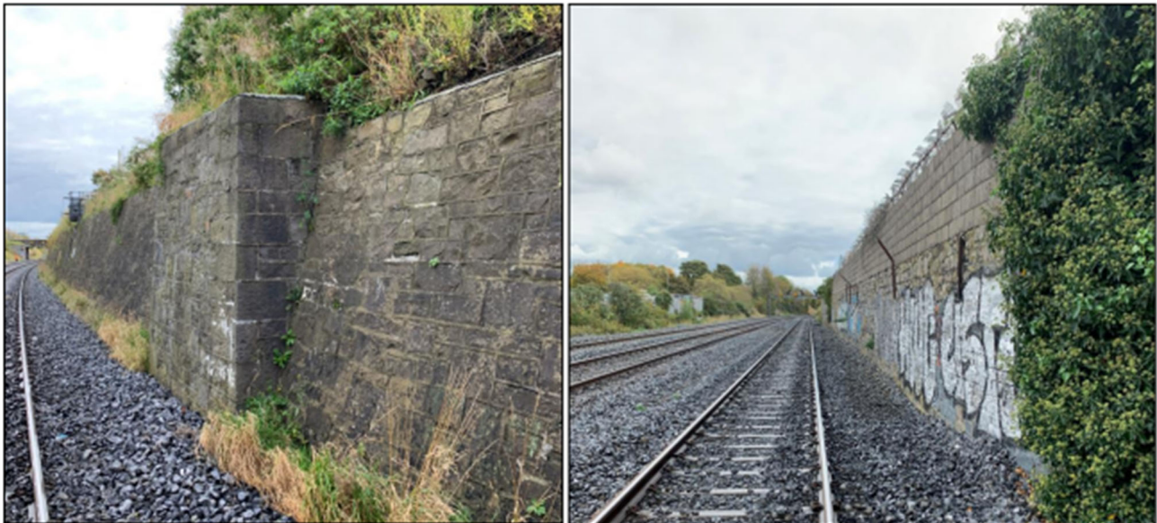
Figure 4-79 Masonry Retaining Wall Buttress and Heightened Wall Sections (Southern Boundary)
