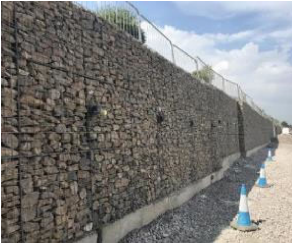
Figure 4-4 Example of Gabion Basket Wall
