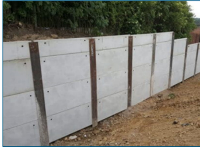
Figure 4-5 Example of King Post Retaining Wall
