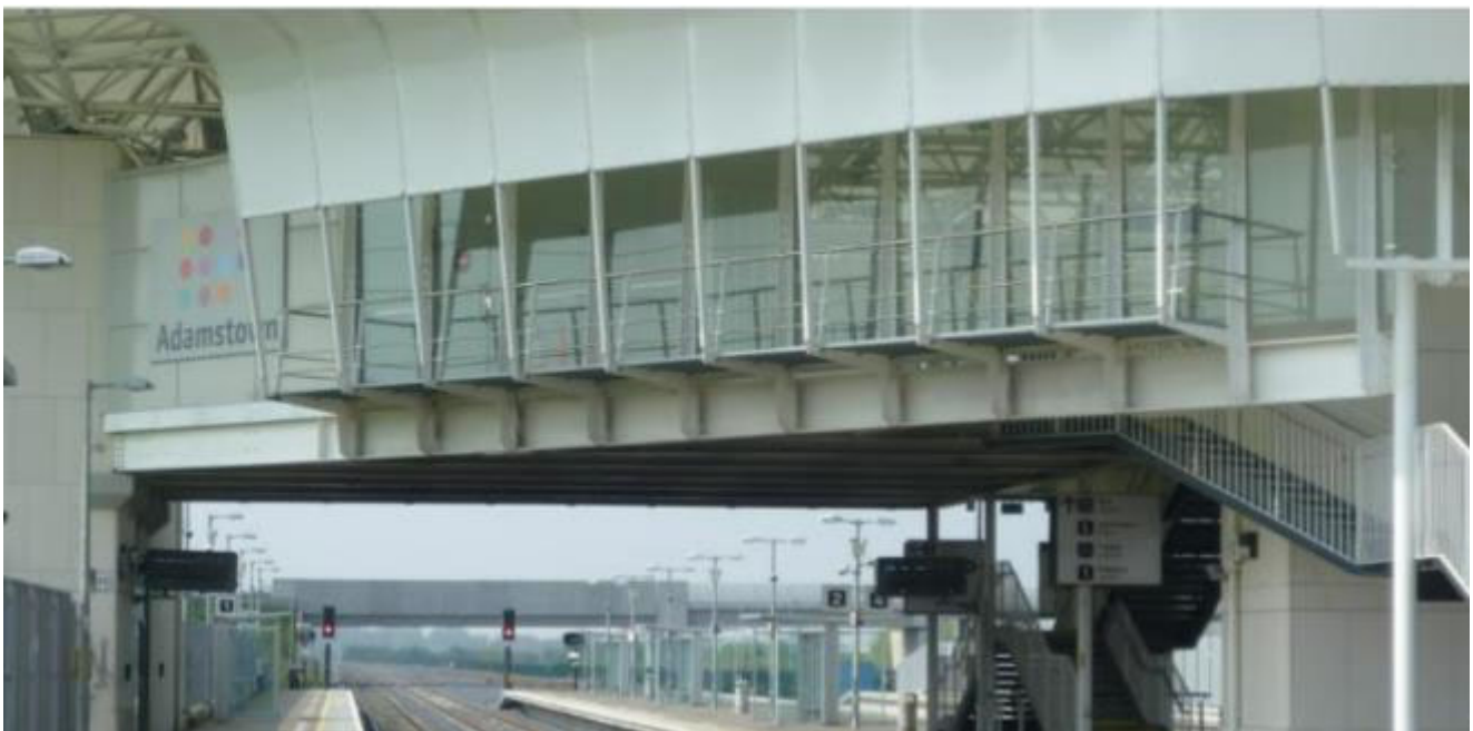
Figure 4-36 Adamstown Station - View of the Maintenance Platform
