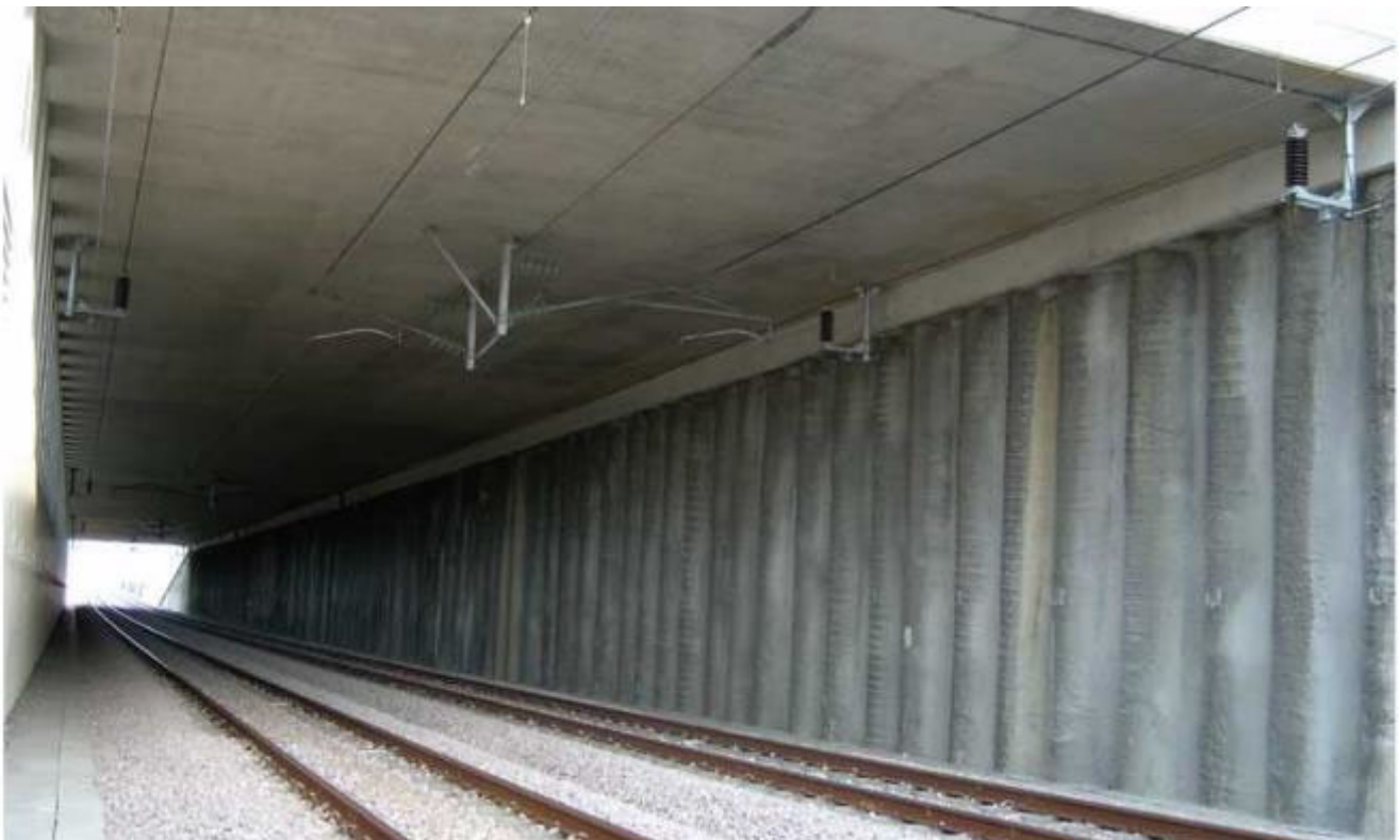
Figure 4-3 Example of a Secant Pile Wall
