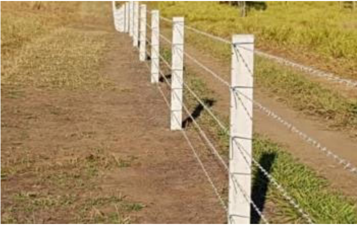
Figure 4-8 Post and Wire Fence
